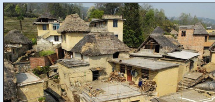
Many houses in China's Yunann province lack sanitation and ventilation systems.
